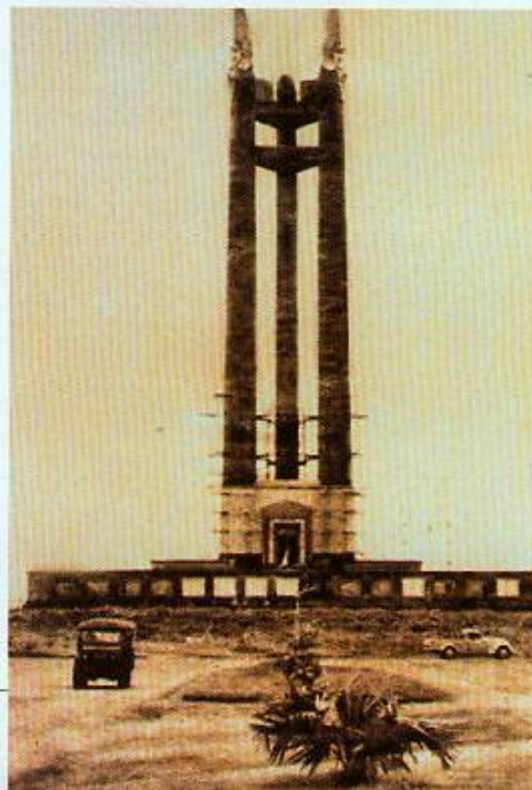
Construction of the pylon of the Quezon Memorial Shrine.
